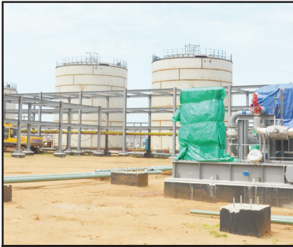
Construction works of Kingfisher Central Processing Facility ready next year Page 23
