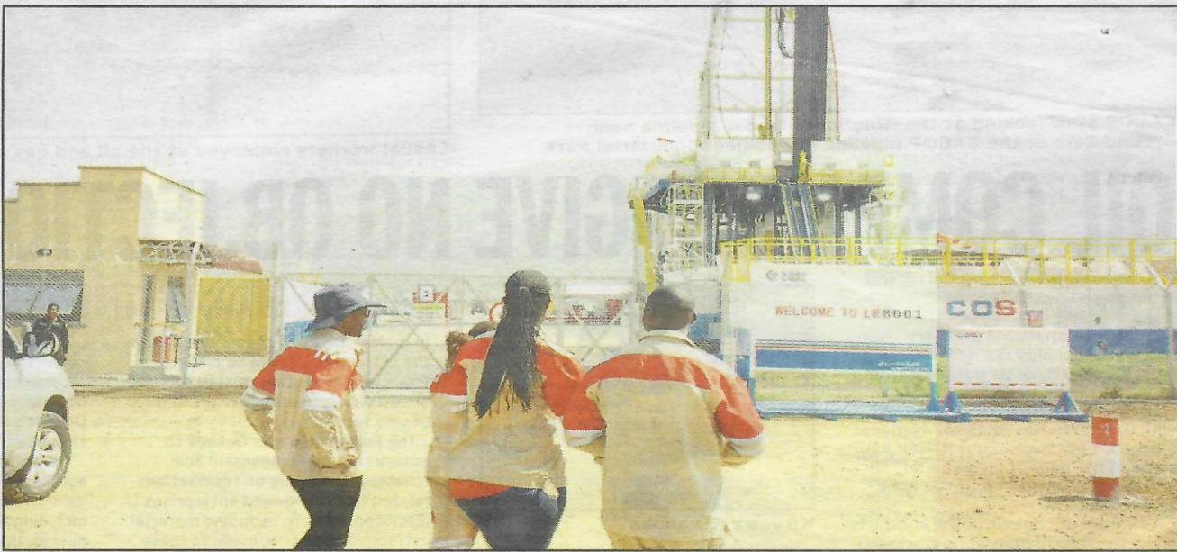
The first oil rig at KingFisher oil field in Kikuube district, Bunyoro sub-region is ready to start drilling oil
